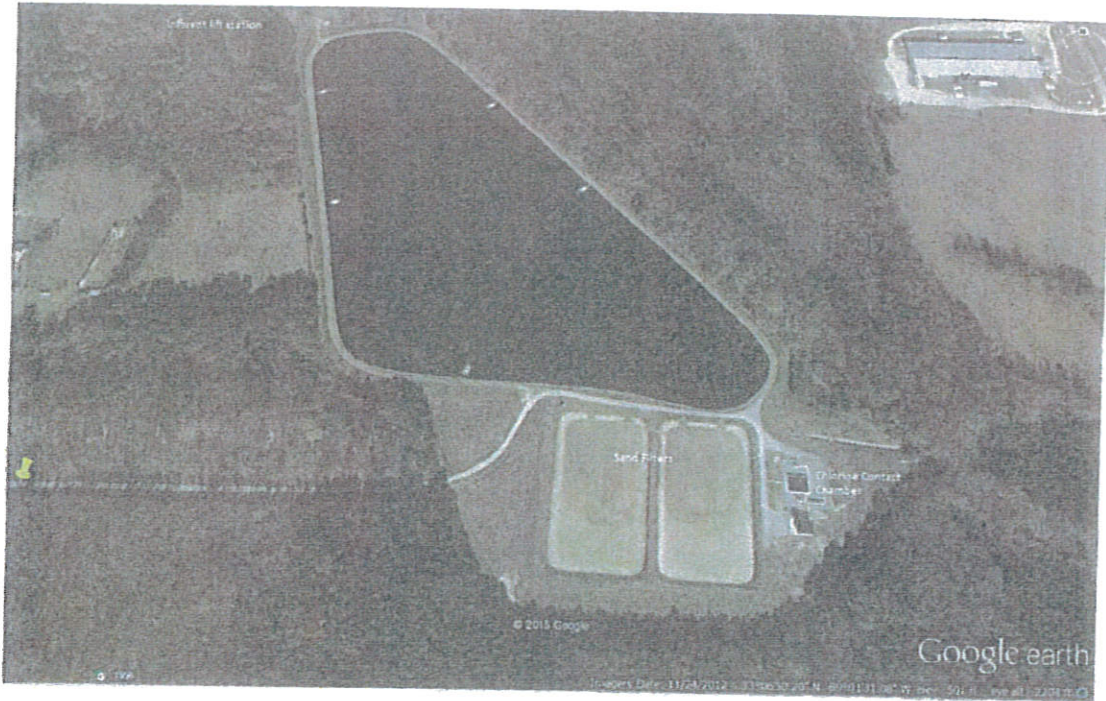
Louisville East POTW facility aerial
