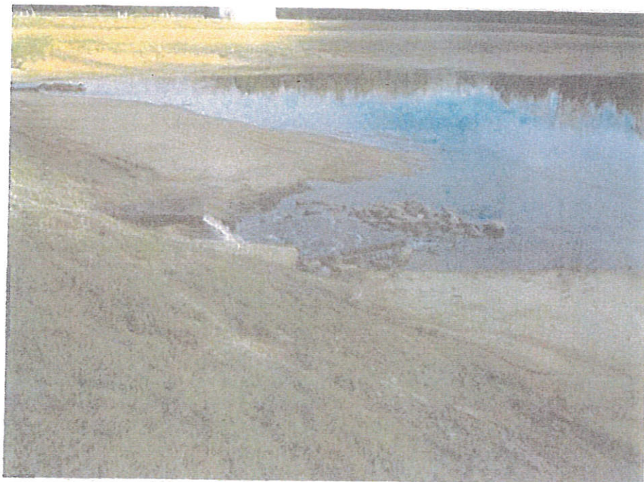
Louisville East POTW; sand filter in 'fill' part of cycle
